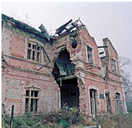
The heavily damaged train station in Vukovar
